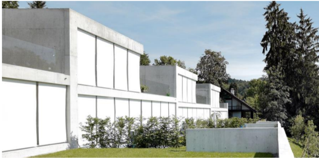
Example of vertical window awnings
